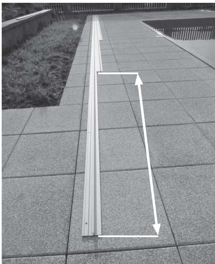
**UK** THE SPACING BETWEEN RAILS CORRESPONDS TO THE LENGTH OF ONE MODULE, FROM WHICH ONE SHOULD SUBTRACT 100 - 150 MM
