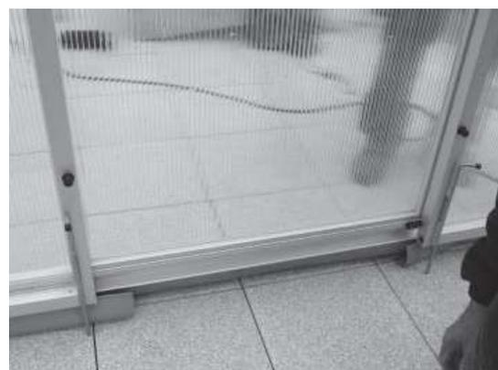
FITTING THE ARRESTING LATCHES OF SILL-FREE DOOR – 2 /
